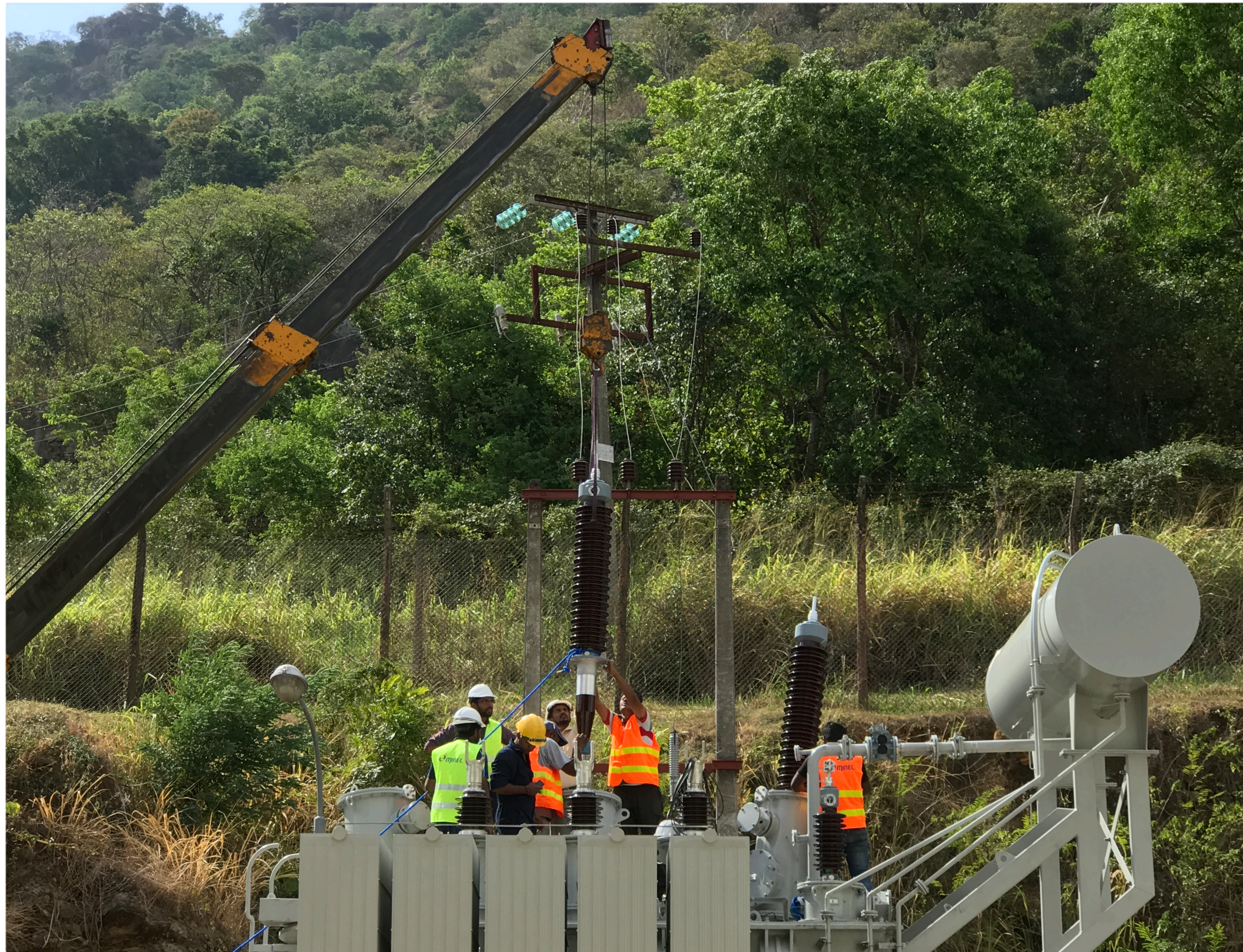
71 MVA, 138/10.5 kV Generator Transformer Project at Samanalawewa Power Station
