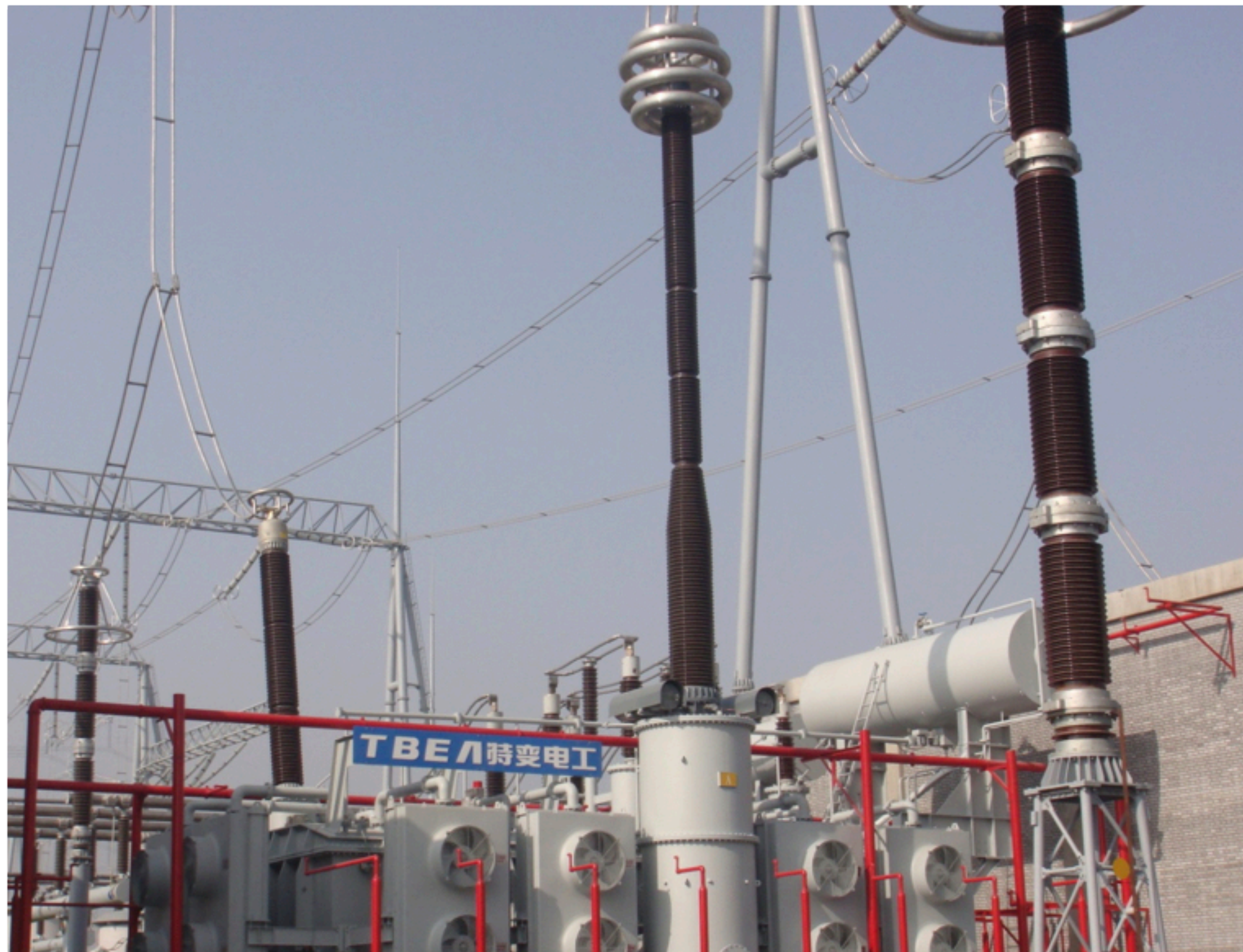
220 kV Transformers with TBEA to Victoria PS, Samanala PS, Kotugoda GSS
